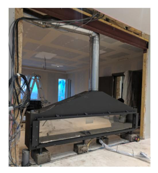
Now create a frame for the enclosure. Use only non-combustible materials, such as aluminium or steel stud frame. Below image shows the installation of a simple 'up and out' flue and the construction of a TV recess:
