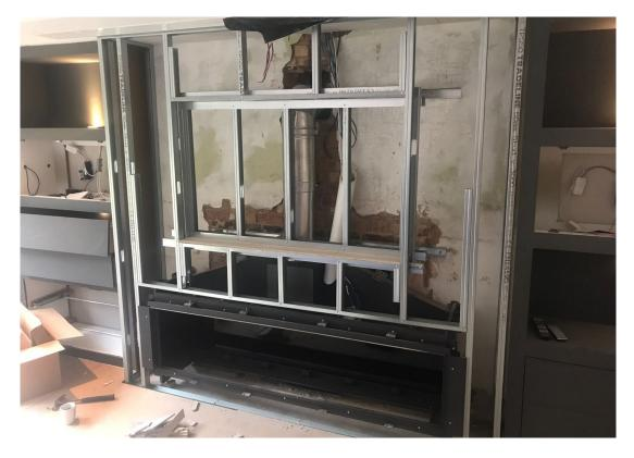
The enclosure should be closed off with two layers of non-combustible fireboard such as PromaFour, Supalux or Glassroc. Do no use simple plasterboard. Protect the TV recess with the same materials.
